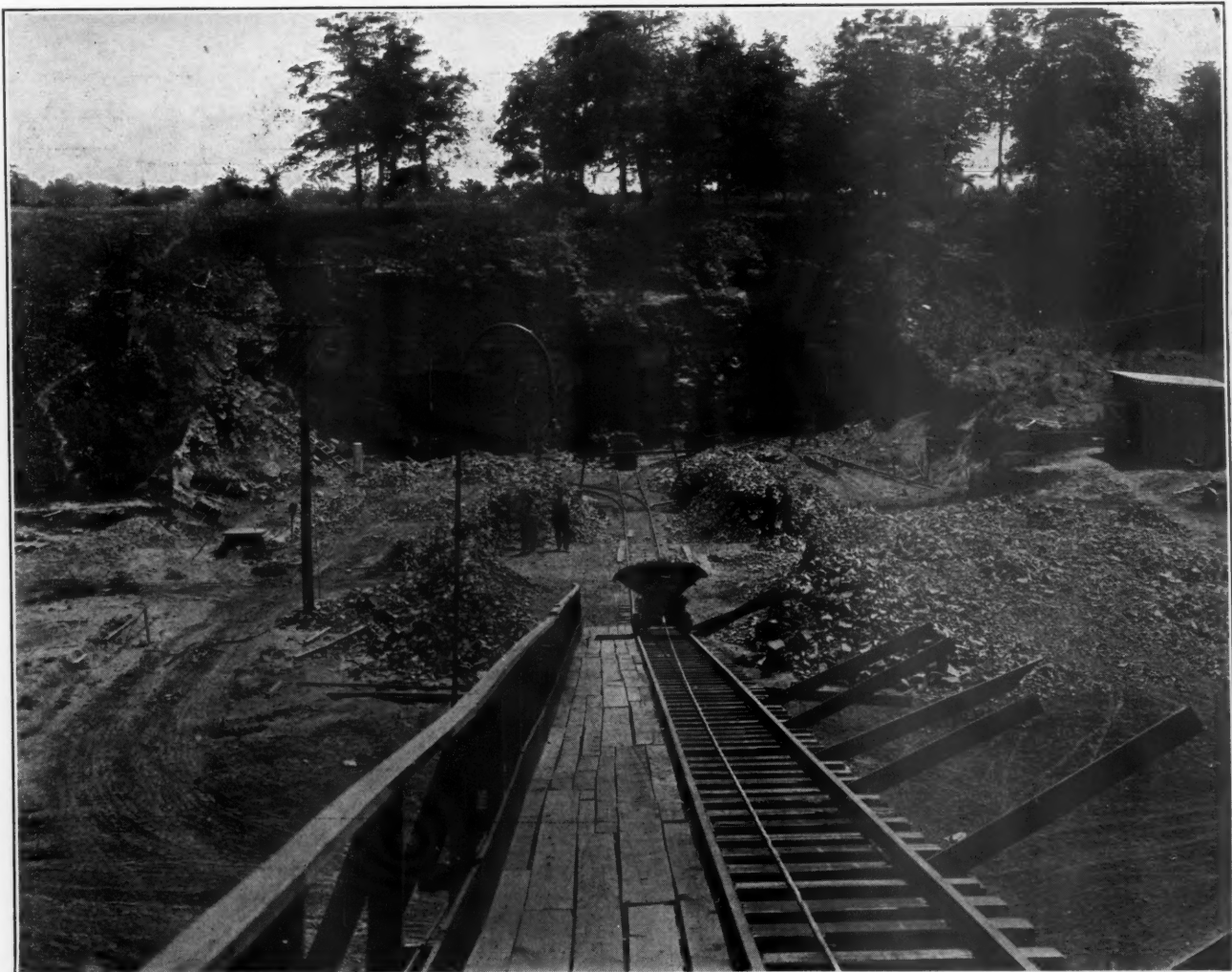
View from top of incline showing entrances to quarry.
